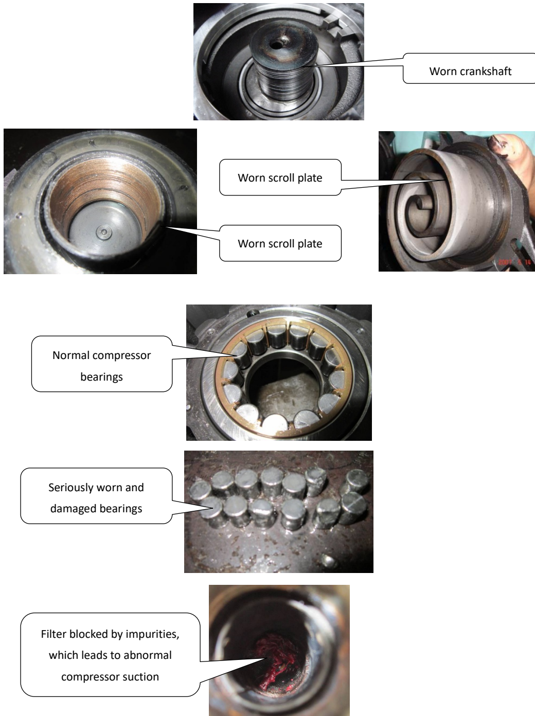
Figure 6-2.11: Effects of spoiled compressor oil
