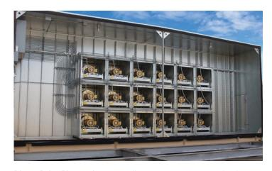
**Direct-Drive Plenum** fan arrays allow up to 100 percent redundancy for greater systems reliability and up to 10 percent increased efficiency.
