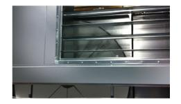
Air-to-air plate heat exchangers are a great solution to recover sensible energy (heat only) from an exhaust airstream, with little or no cross-contamination. These exchangers may also be used for free reheat in dehumidification applications, including dedicated outdoor air systems. Where exhaust air is not available, exchangers can be used in series to heat the dehumidified air.
