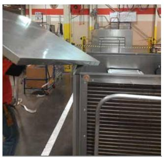
There is gasket along top of the unit at the COU panel and wall panels. The gasket should be in good condition to be reused, but if not, the gasket will need to be replaced. The door flange will have gasket along top and bottom as shown above and not on the top like wall and COU panels.
