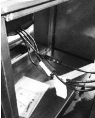
Figure 35. Horizontal section-to-section high voltage quick connects
