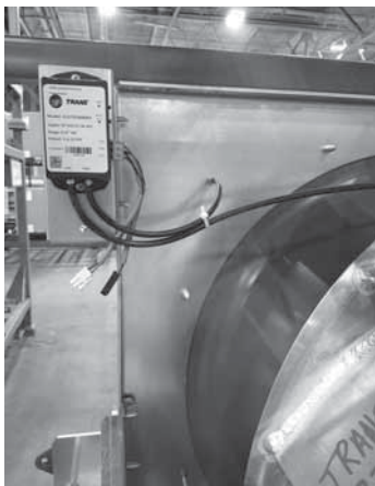
Figure 169. Typical transmitter install for DDP fans
