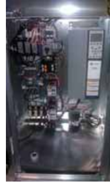
Figure 146. Internally mounted VFD
