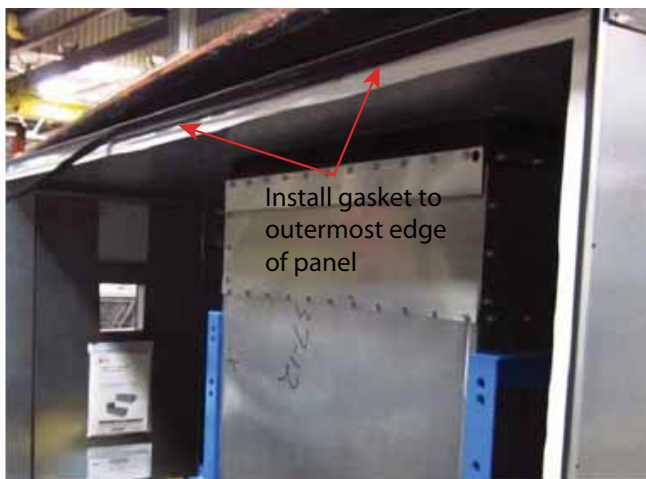
Figure 32. Install gasket to outermost edge of panel
