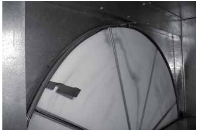
Figure 196. Pull the segment up and out of the wheel frame to remove
