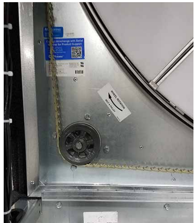
Figure 171. Confirm proper belt tracking on wheel rim
