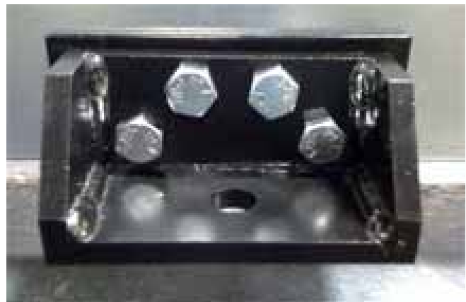
Figure 71. Seismic anchor
