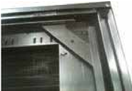
Figure 28. Coil structural gusset
