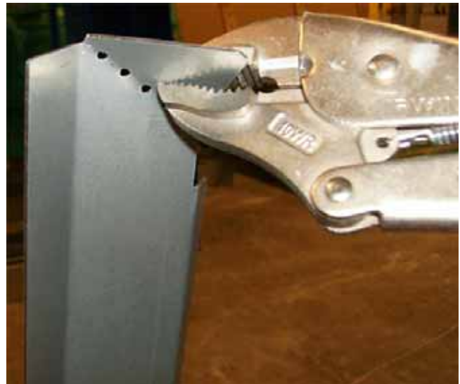
Figure 59. Bend end tabs, apply Butyl tape to flashing
