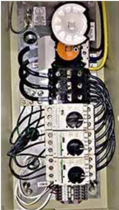
Figure 148. External motorized impeller control panel (MICP)
