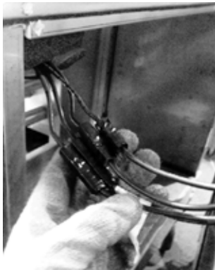
Figure 36. Horizontal section-to-section high voltage quick connects
