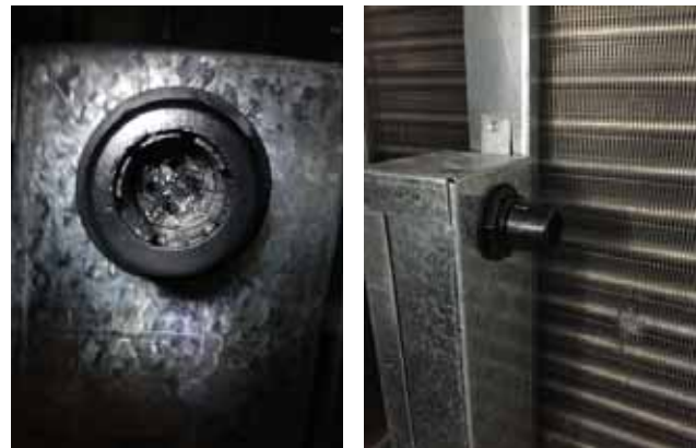
Figure 207. Plug pins into socket, then tighten compression nut
