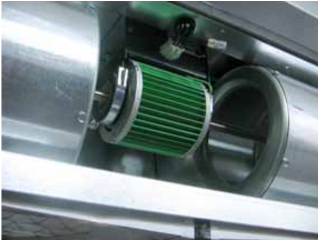
Figure 107. Motor attachment screws are behind motor
