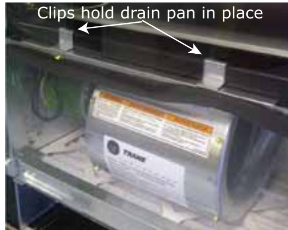
Figure 101. Clips hold drain pan to the fan board
