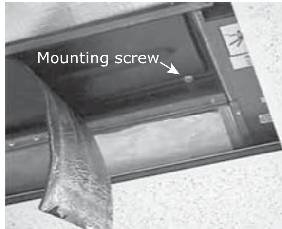
Figure 100. Peel insulation back to see mounting screw
