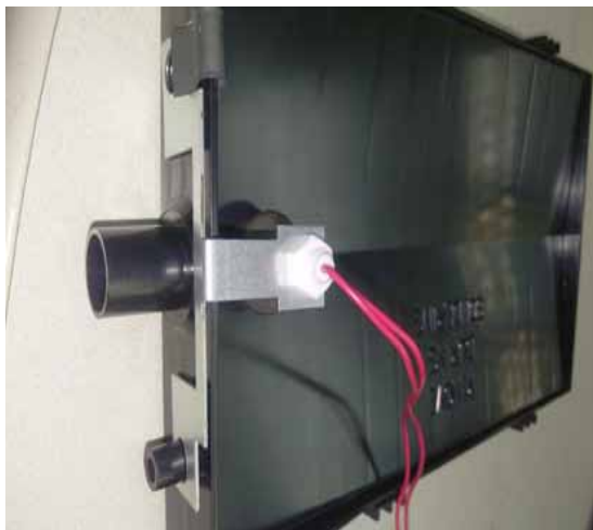
Figure 28. Condensate float switch installed in horizontal auxiliary drain pan
