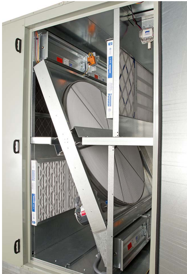
Figure 60. Total-energy wheel module
