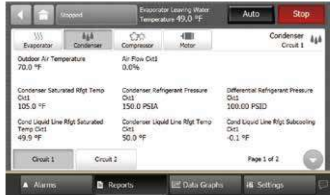
Figure 30. Report condenser screen
